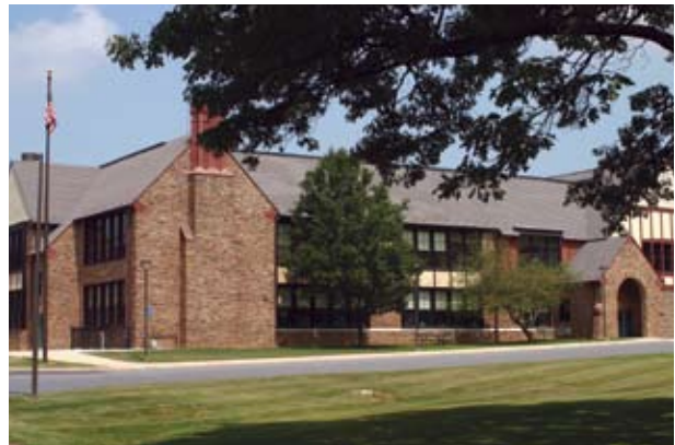
The 1929 Brecht Elementary School was renovated and enlarged in 2000.
