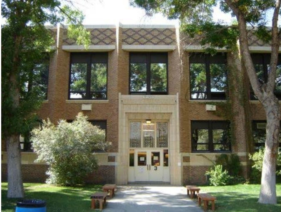
East Junior High of Rock Springs was demolished in 2012. (photo courtesy Mary Humstone)
