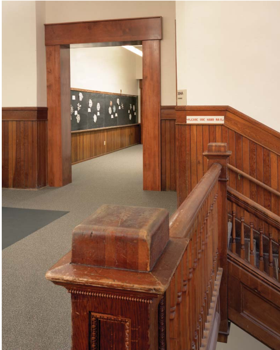
Woodwork in Historic School Building Before Refurbishing
