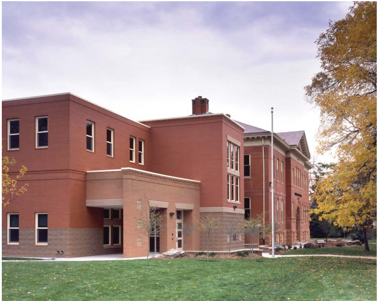
New Entry Addition Connected to Historic 1906 School Building
