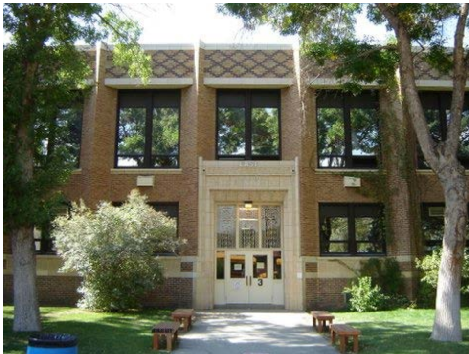
East Junior High of Rock Springs was demolished in 2012. (photo courtesy Mary Humstone)
