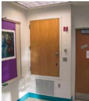
Each classroom in the three schools has its own heat pump in a closet for individual heating and cooling.
