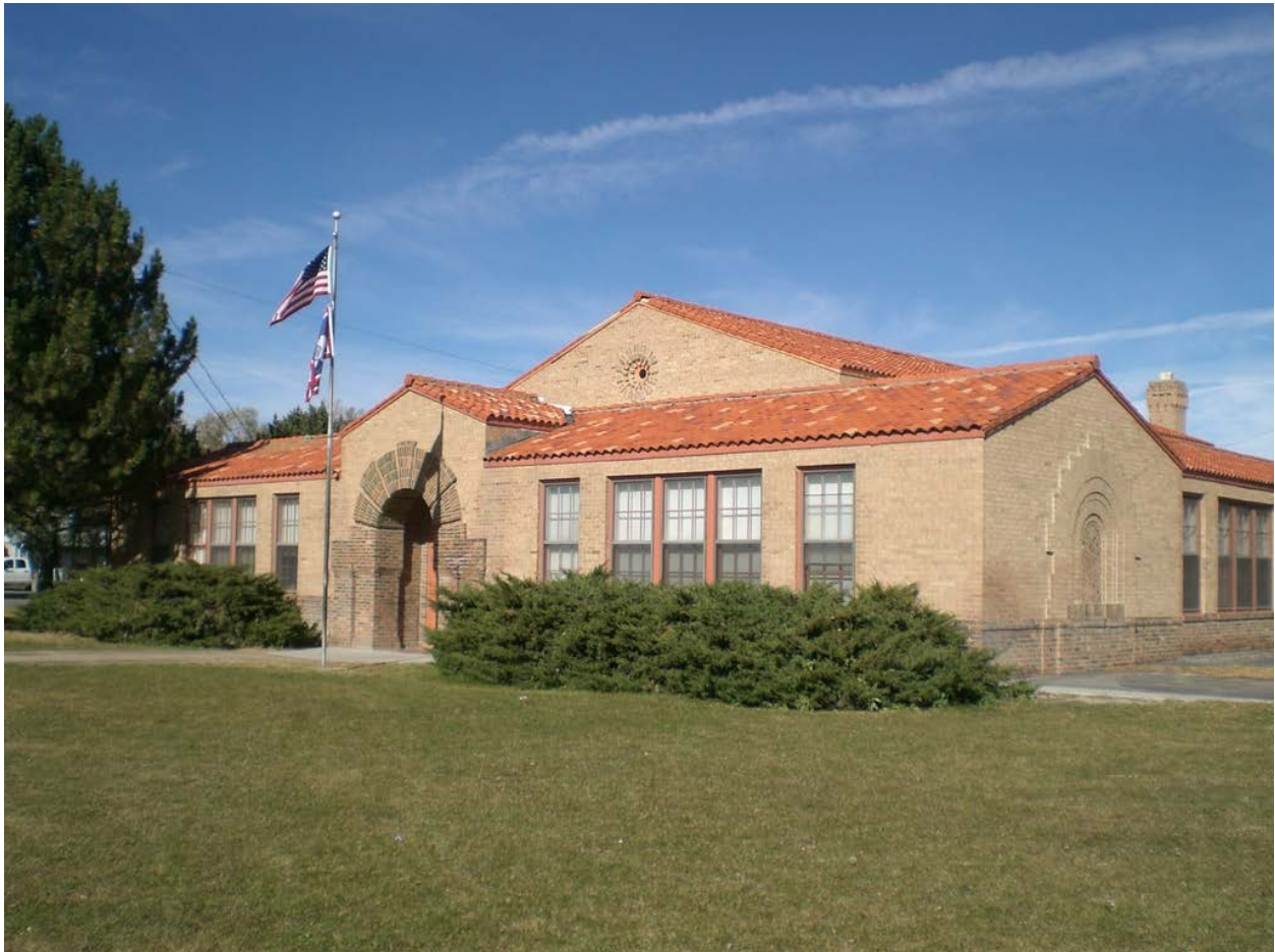
Sinclair Elementary School in Sinclair is poised to undergo a $1.7 million renovation. (Photo courtesy Mary Humstone)
